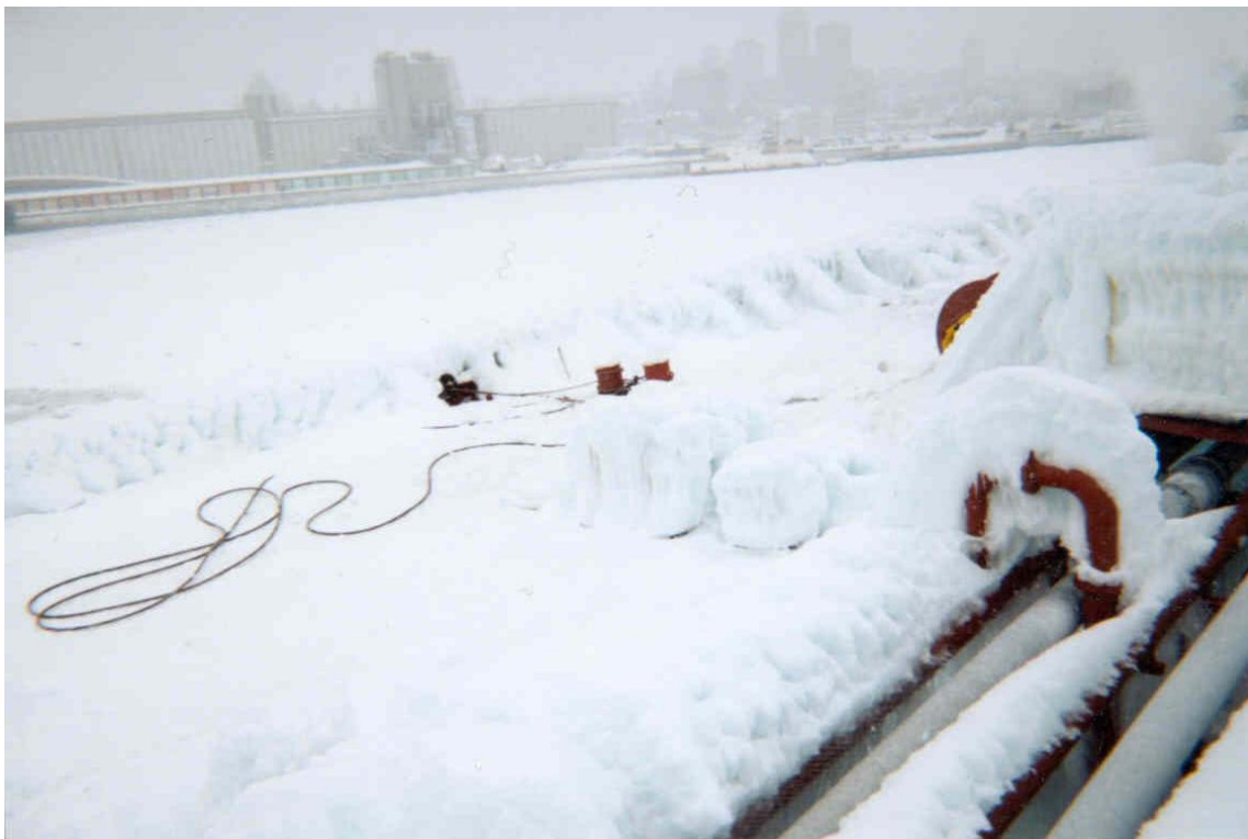
Figures 5.3F– Deck, piping and valves inaccessible
